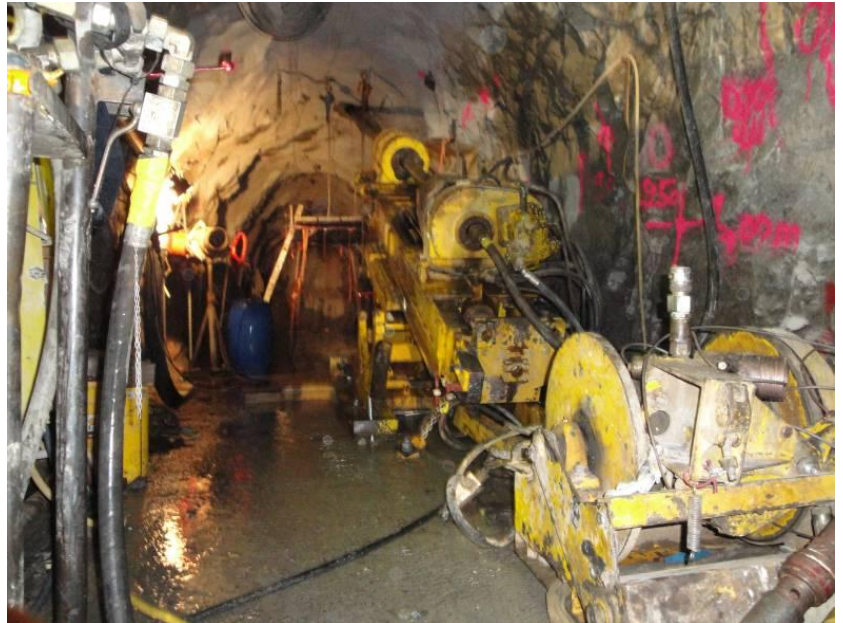
Figure 3: Drilling inclined holes into the roof posed no problem.
