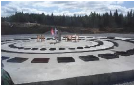
Figure 3: 17.08.2010: completion of the drilling base
