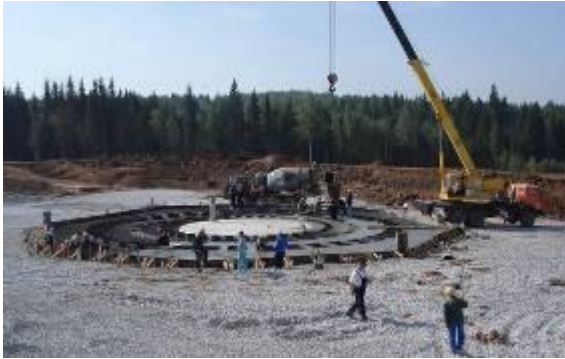
Figure 2: 16.08.2010: constructing the drilling base for the skip shaft
